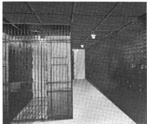
INTERIOR OF VAULT—SHOWING BANK'S PRIVATE SECTION, AND SAFETY DEPOSIT BOXES
